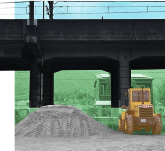
JR (Japan Railway) Kosei-Line (1974) A north-south elevated railway. At 12m high, it maintains a permeable ground plane, crossing over roads without conflict.
